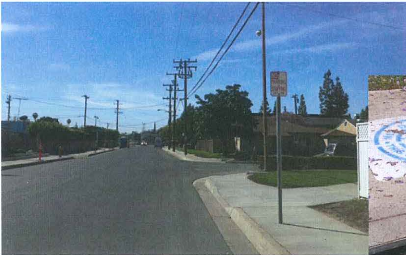
New Asphalt Overlay on Bradbourne
