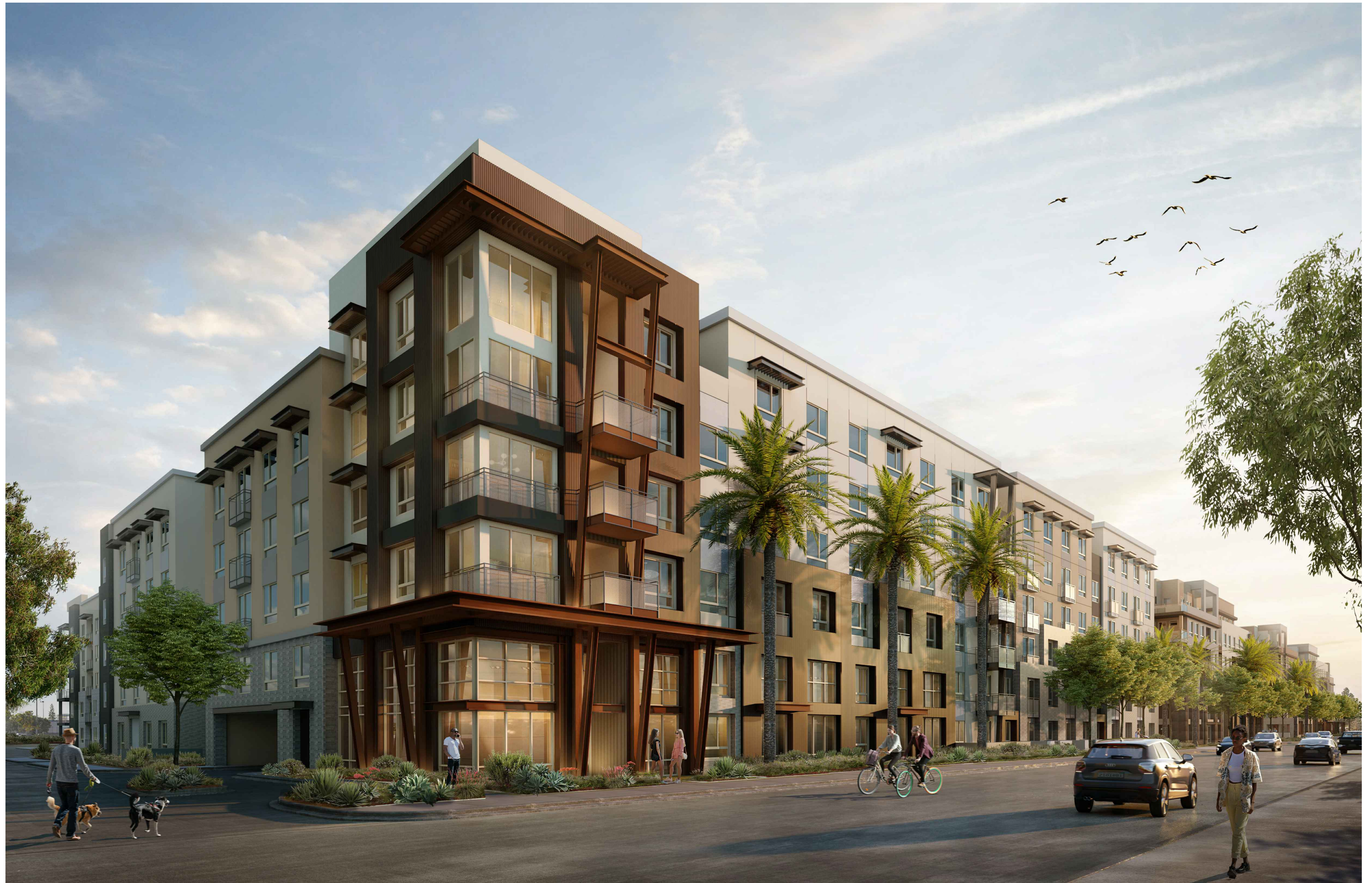
BUILDING B - VIEW OF NORTHEAST CORNER
