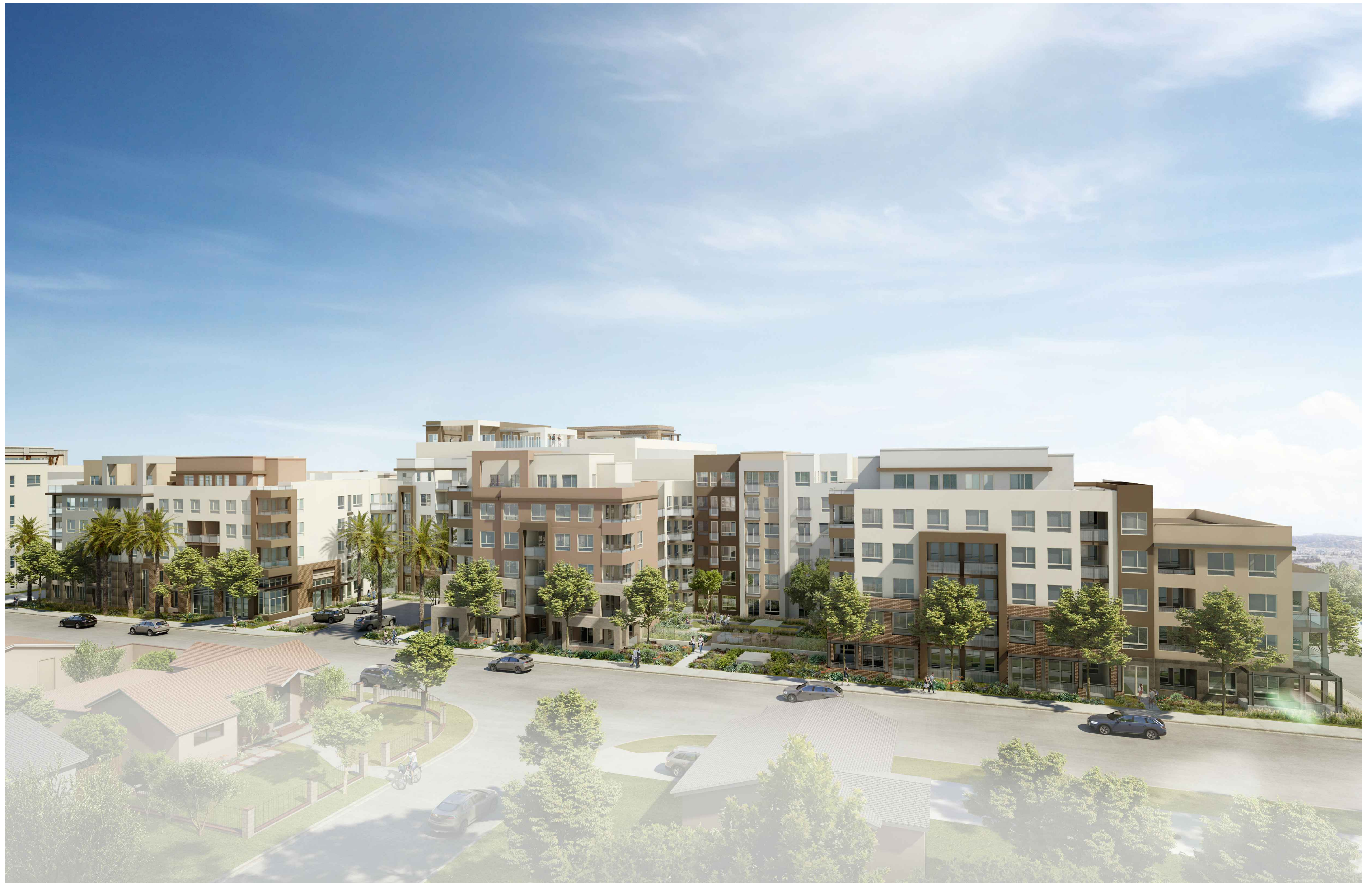
BUILDING A - VIEW OF BUSINESS CENTER DR. ELEVATION
