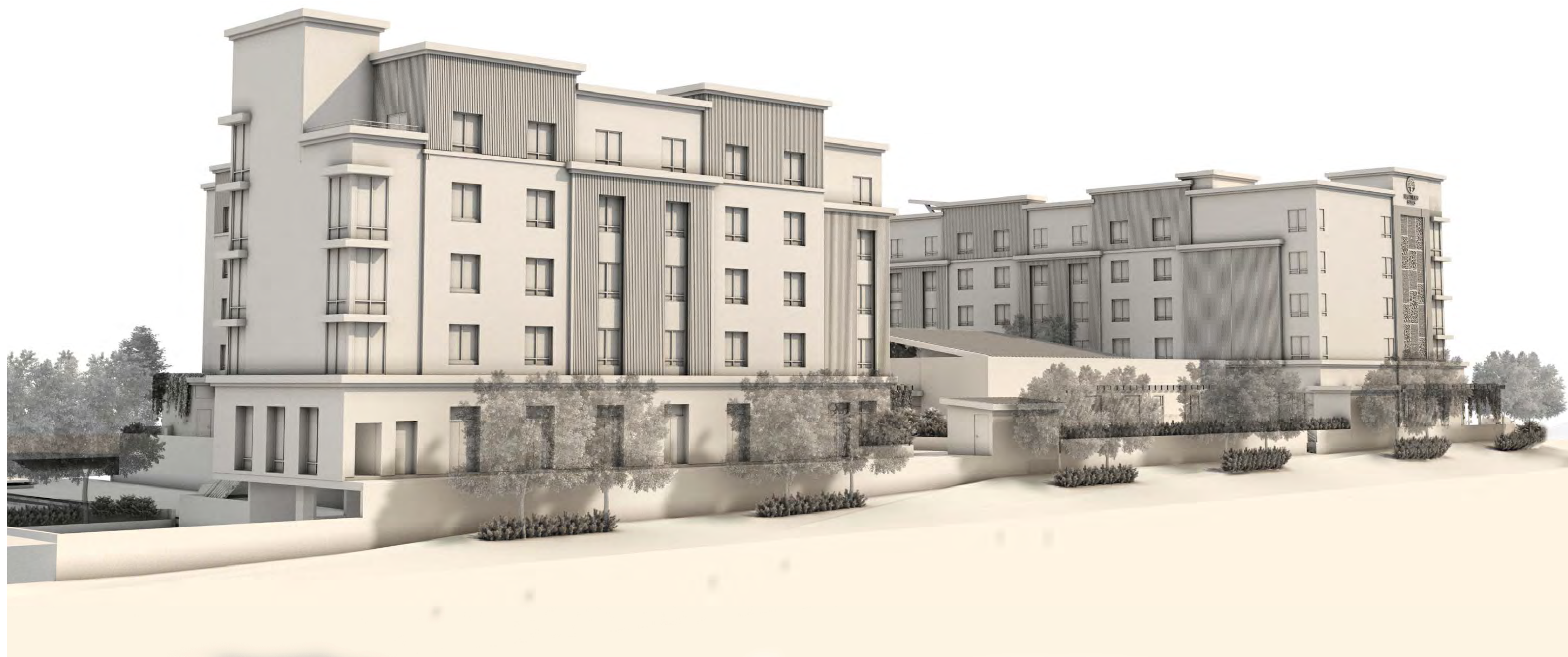
PERSPECTIVE VIEW FROM SOUTHEAST CORNER LOOKING NORTHWEST
