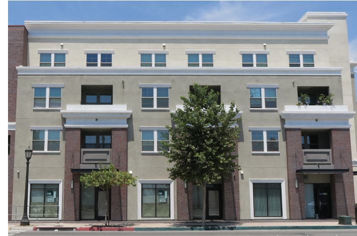
The Huntington Apartments (1413 Huntington Drive), Duarte. Stepping back of the top floor of the building to reduce massing closest to the pedestrian frontage.
