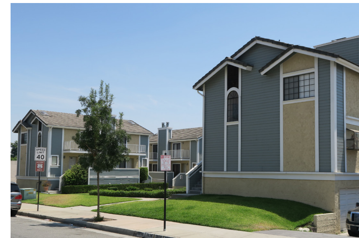
Lack of relationship between units and frontage
