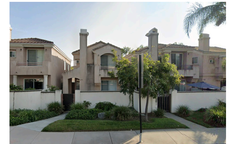
Lack of weatherproofing of exterior materials
