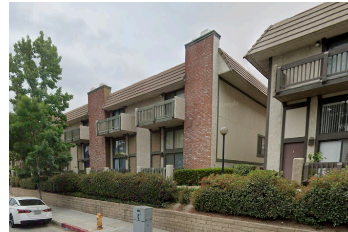
Older apartment building in Duarte
