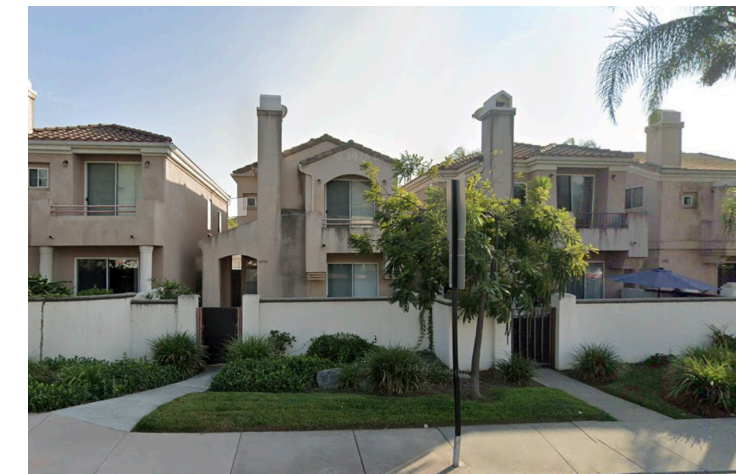
Lack of weatherproofing of exterior materials
