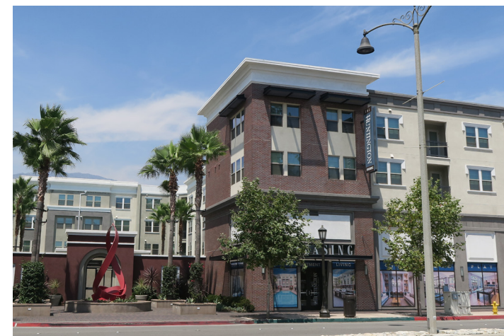
New mixed use project in Duarte on Huntington Drive, The Huntington at 1413 Huntington Drive
