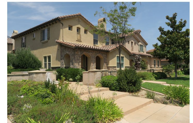
Survey of multifamily residential buildings in Duarte
