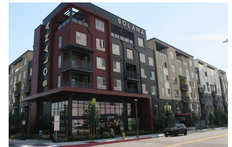
New high density multifamily project in Duarte, Solana at 1750 Fasana Road
