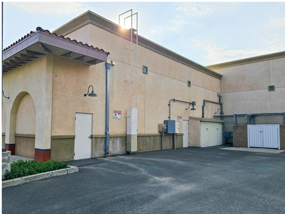
North Wall of Tenant Space (Behind Building)
