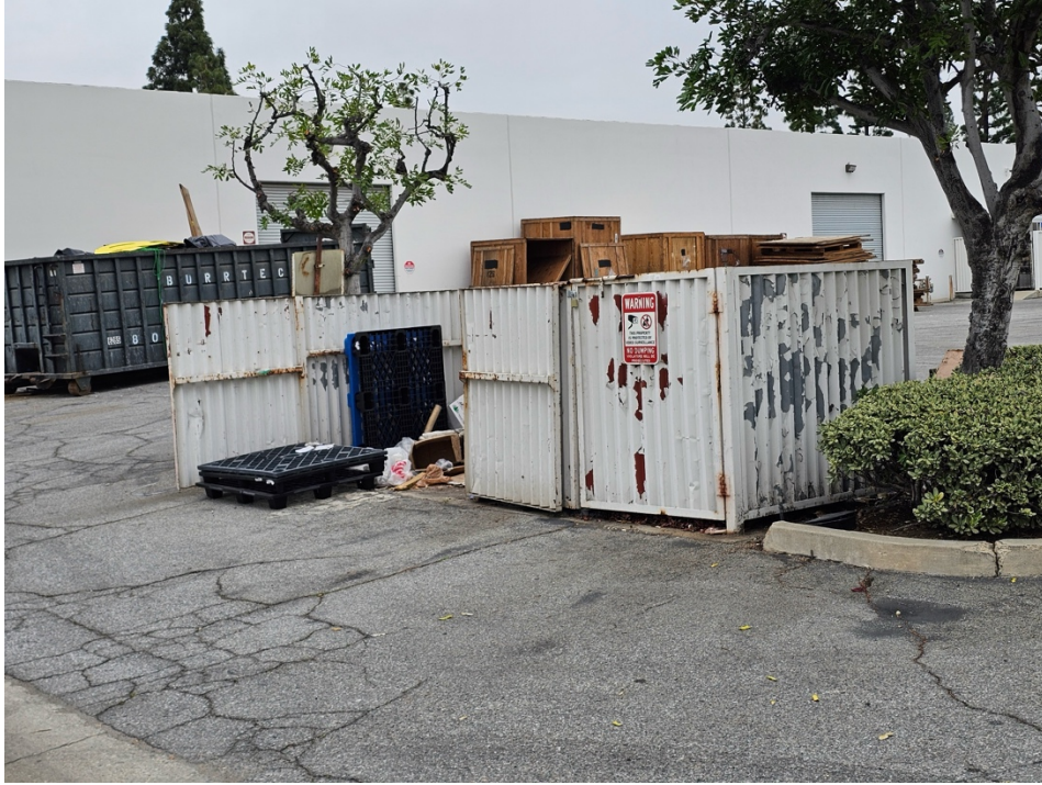
Existing Trash Enclosure
