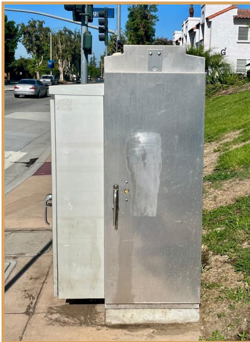
East (Side-Traffic Controller)
