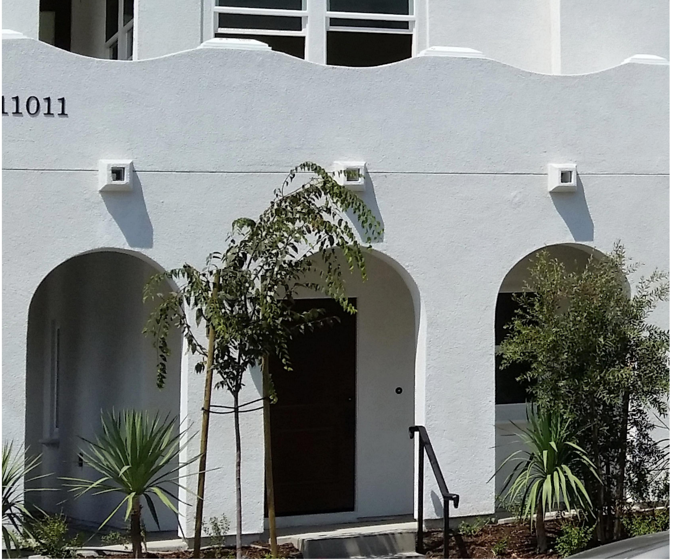
8. STUCCO ARCH AT ENTRY
