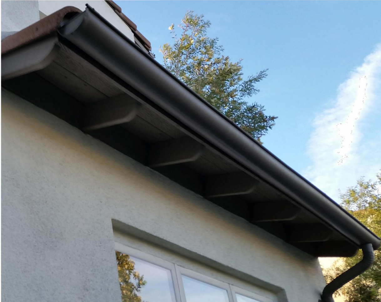
13. EXPOSED DECORATIVE TRUSS TAILS W/ EAVE BOARD & GUTTER
