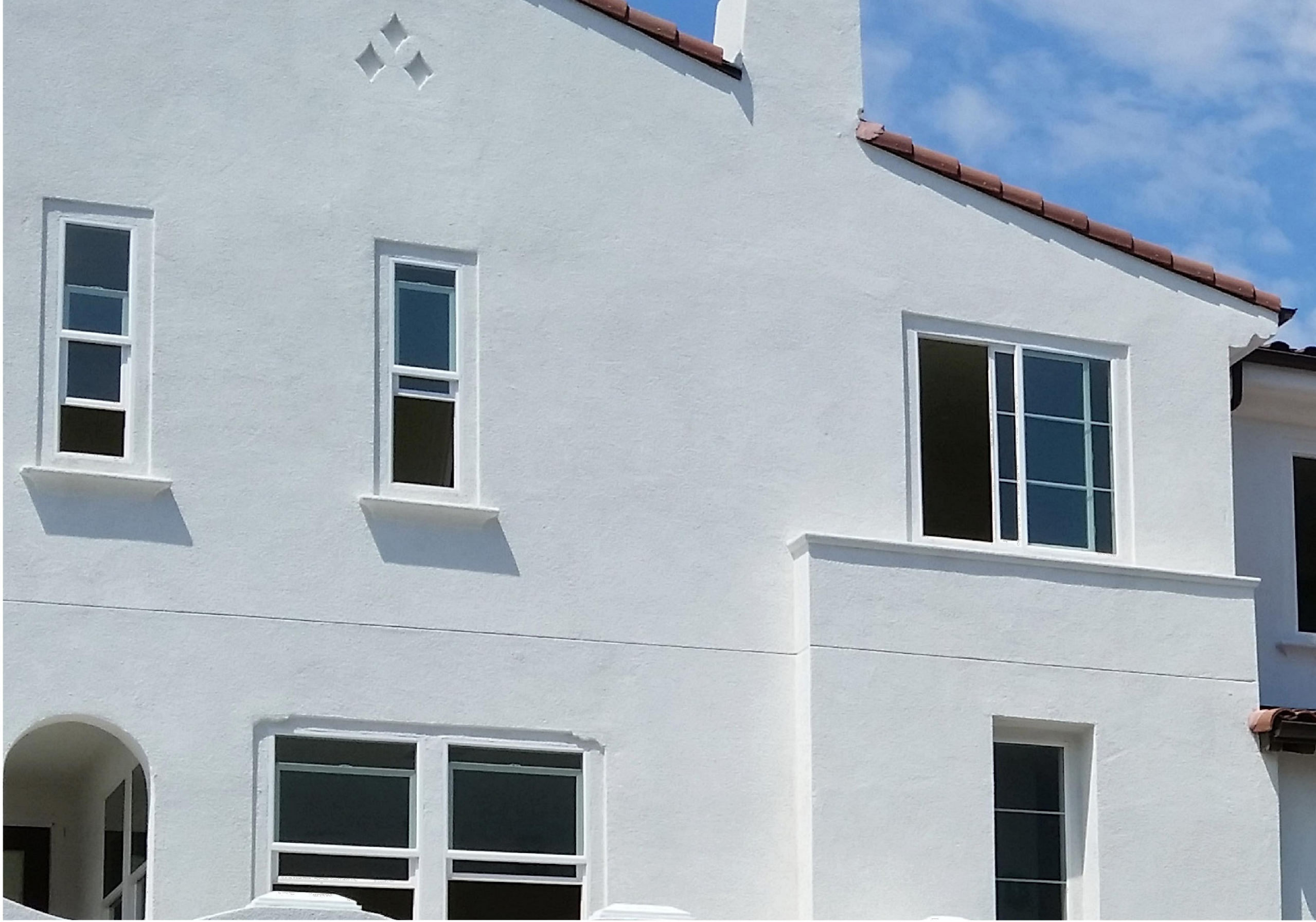
6. DECORATIVE STUCCO SCALLOPED SILL TRIM & SHELF
