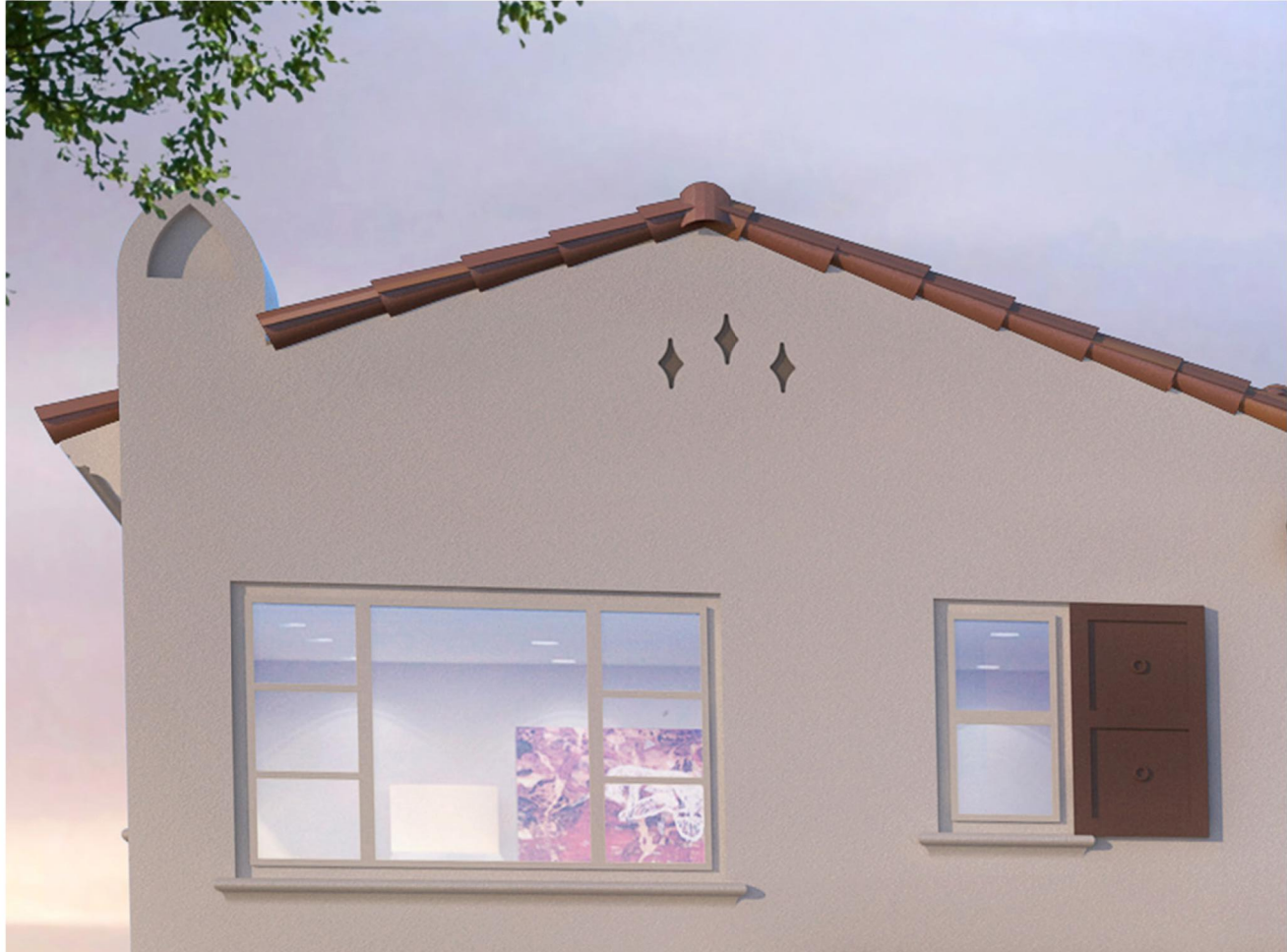
9. STUCCO FINIAL & GABLE END FAUX VENT RECESS
