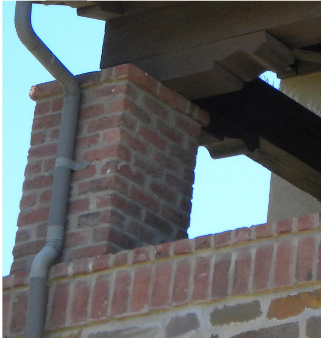
12. BRICK COLUMN & WOOD BEAM
