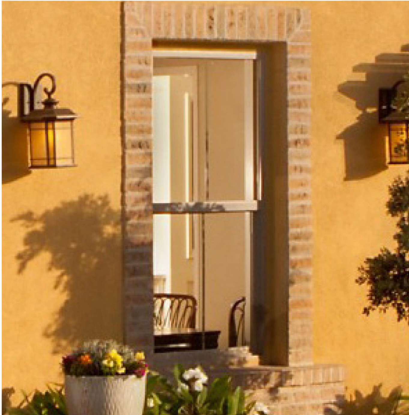
9. BRICK VENEER HEADER & SILL TRIM
