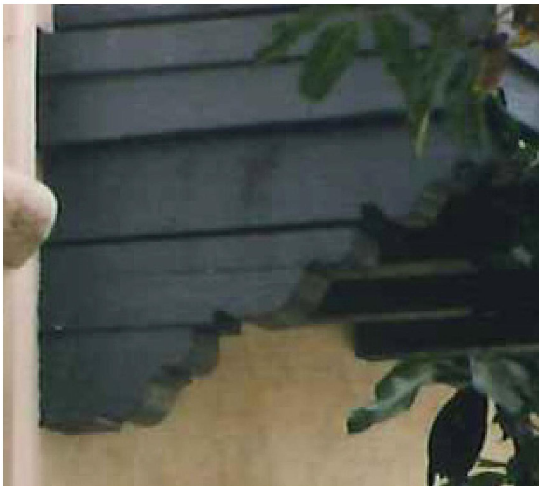
2. CORBEL OUTLOOK AT AWNING
