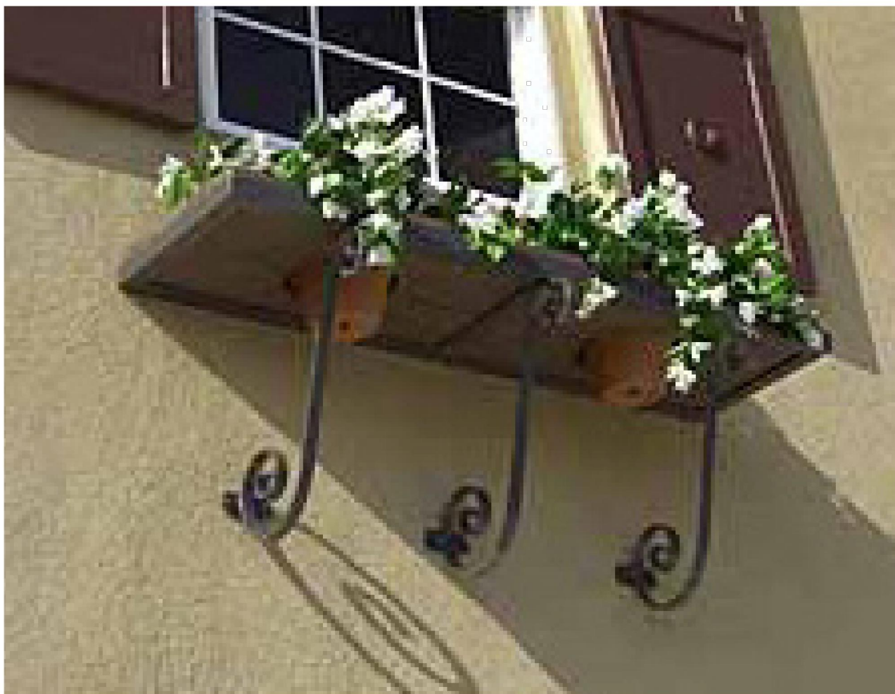
1. WOOD POT SHELF W/ METAL SCROLL BRACKETS
