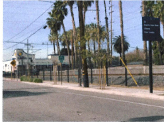
Duarte Rd at Buena Vista: new sidewalk, pedestrian lighting, landscaping and wayfinding
