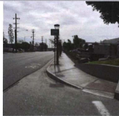
Highland Ave at Evergreen St: new ADA curb ramp, sidewalk, bike route sharrow
