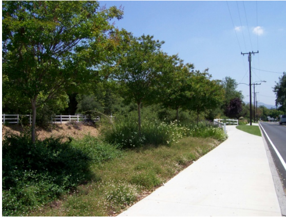
COMPLETED ROYAL OAKS PEDESTRIAN IMPROVEMENTS
