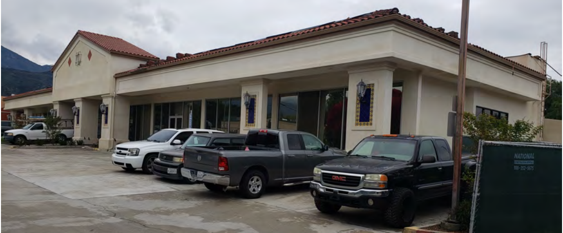
Unit at rear of 4-unit building that school proposes to occupy.
