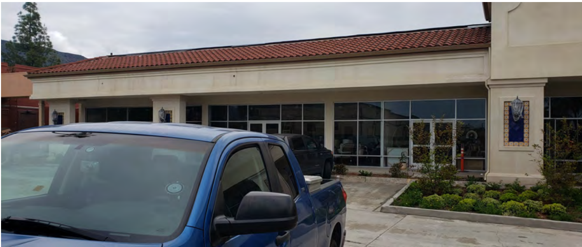
Vacant units of 4-unit commercial building
