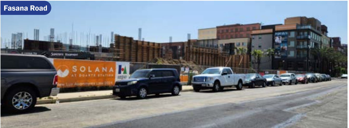
Duarte\City of Hope Station - Highland Ave. Entrance
