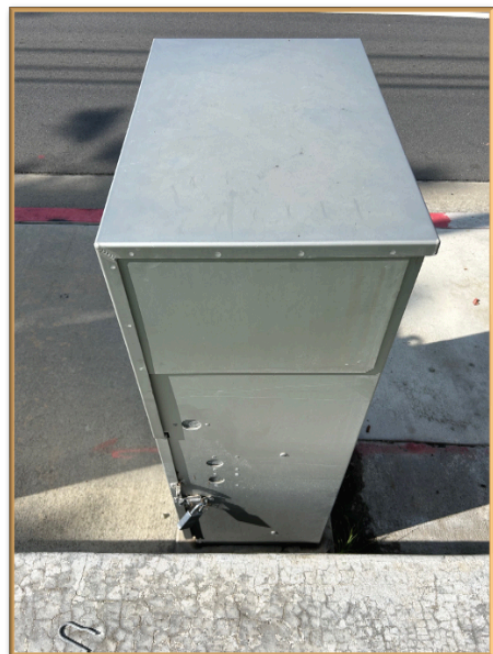
East (Back of Pedestal)
