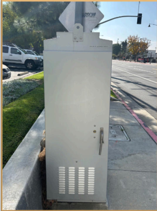
North (Side of Utility Box)
