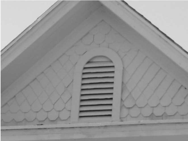
East facing Front of house 2003-01-17 / 1017 Oak 008.jpg
