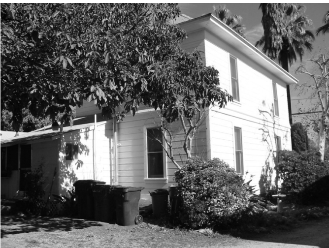
South Rear view of house 2003-01-17 / 1017 Oak 013.jpg
